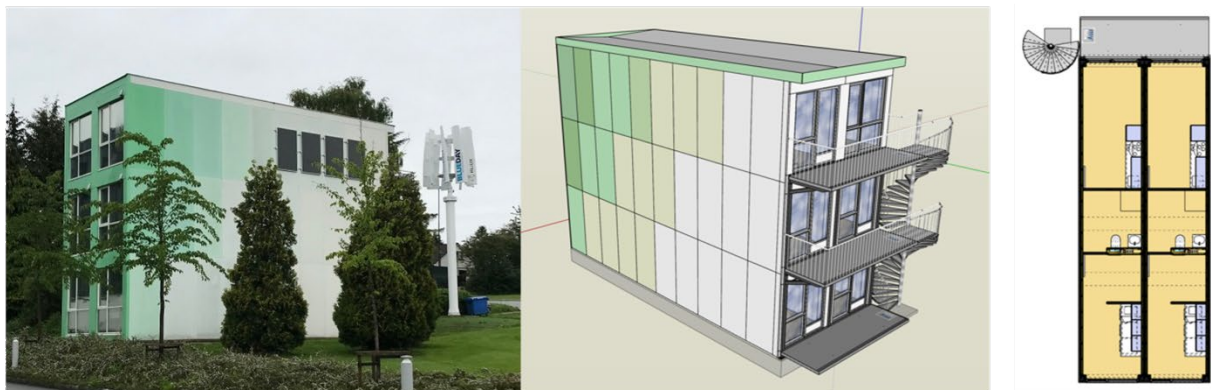
Figure 1: A) A photo of the exterior of the MyBox lab. Towards the right of the building, there are four east-facing PV panels. On the right side is a 3kW VAWT (Photo by H. Syse). B) A building information model (BIM) model used to create the BPS model. C): Overview of the interior of the apartments. BIM model and figure by (Sørstrønen, 2013).
